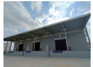
The first Japanese-quality hazardous materials warehouse in Vietnam
